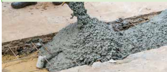
Wet concrete being poured onto steel reinforcement bars at a construction site © Shutterstock
