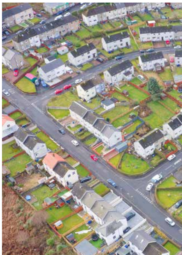
Council flats in a housing estate in Port Glasgow, Scotland, UK © Shutterstock
