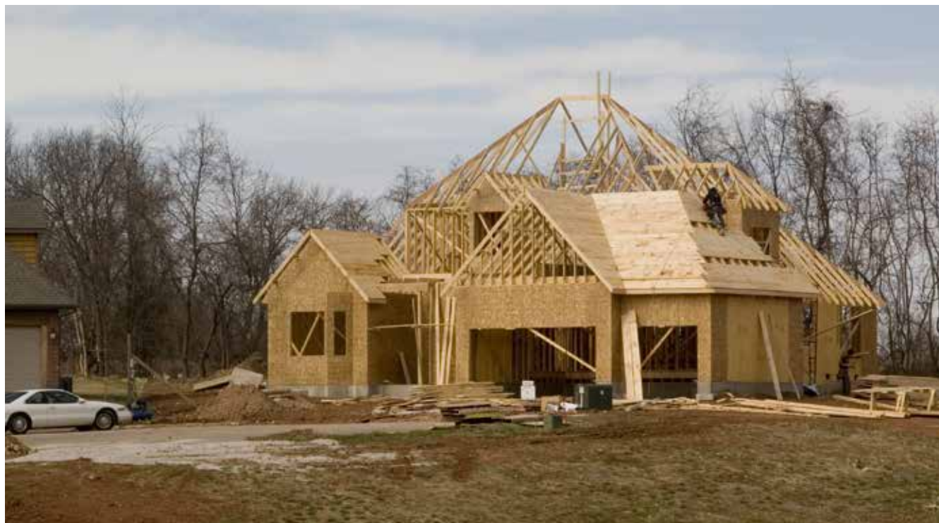
A new home under construction © Shutterstock
