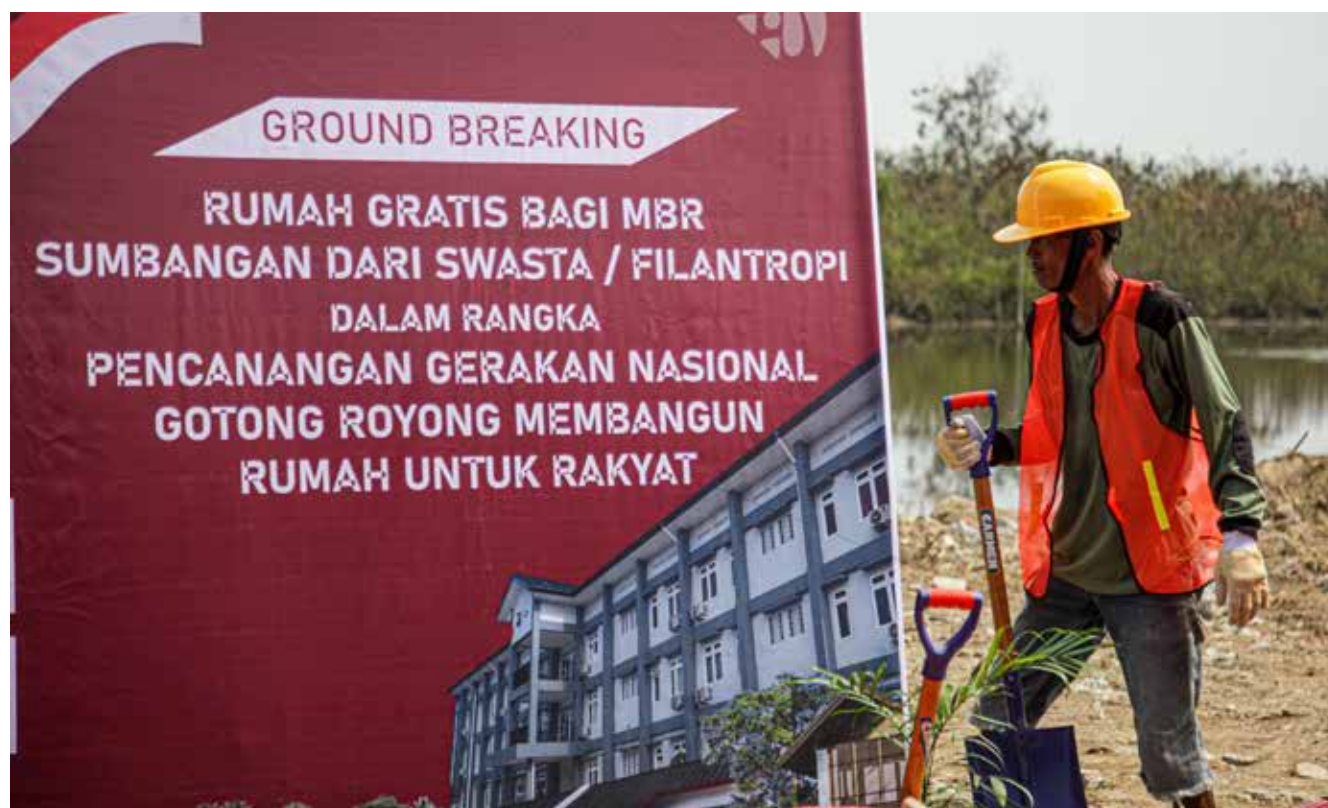
A construction worker at the site of free houses for the poor, which is a government program in Tangerang, Indonesia © Shutterstock
