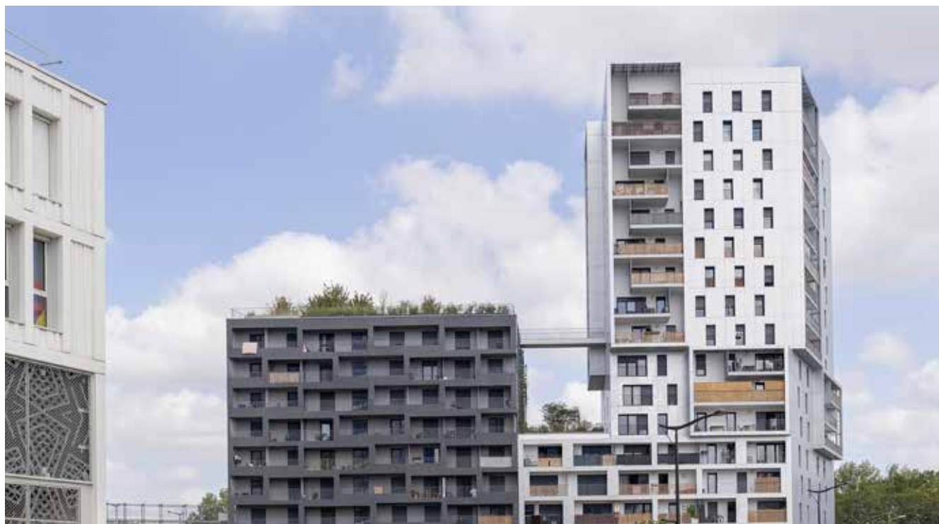
View of a mixed-use real estate complex, housing and shops, built in 2020 in the ZAC Paris Rive Gauche © Shutterstock
